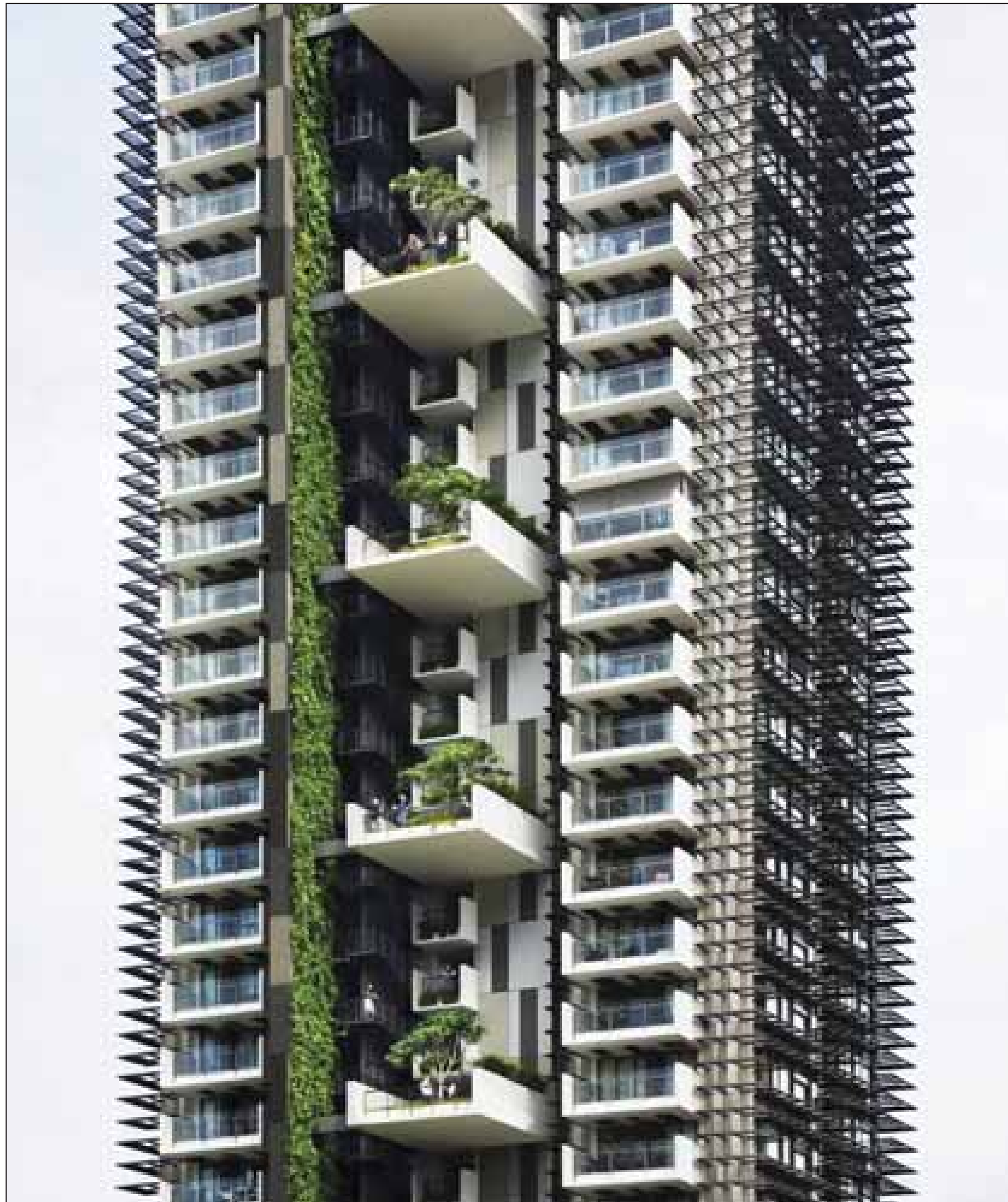
Community sky-gardens, each with a frangipani, protrude from the facade. A green wall of thunbergia rises alongside the fire stairs for the full height of the apartment block – Newton Suites.
