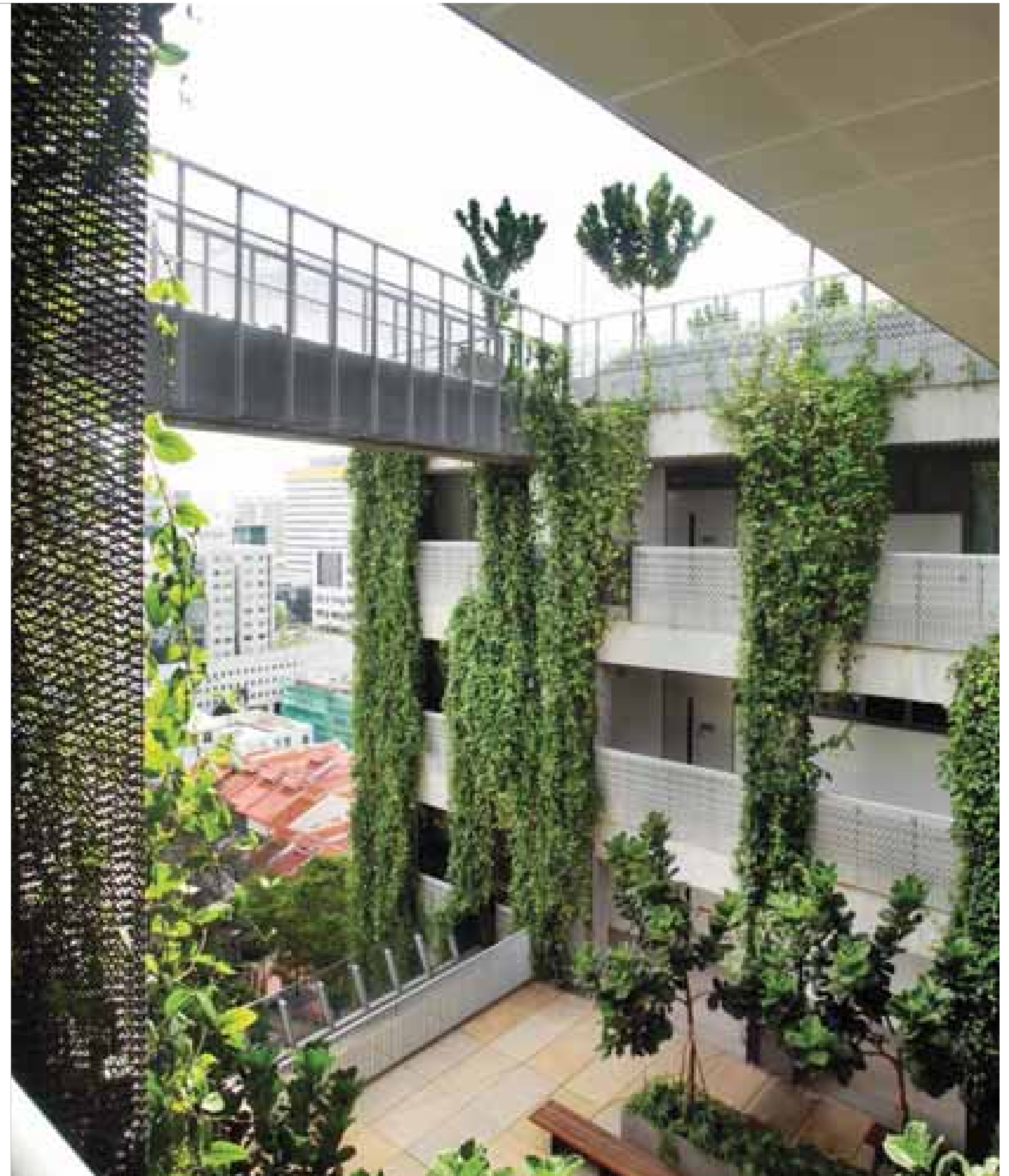
Vast breezeways along the entire building can be seen as a giant wind-catching machine. – School of Arts, Singapore.
