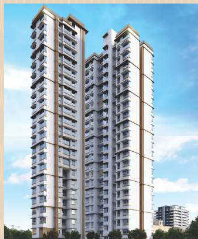
Unity Towers - Worli
